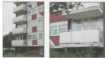
Big Green to be fitted to cover off upper balcony area. Existing safety rail to be removed. Existing windows and doors to remain.
