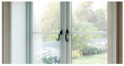
In the UK where external shutters are rare, the vast majority of casements open outwards. Within casements, there are various styles. A flush casement is simply one where the opening window sits flush in its frame, rather than standing proud.
